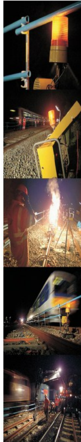
Barrier set at 6ft 6" (2m) from running rail for lines speeds over 100 mph
